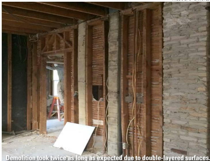
Demolition took twice as long as expected due to double-layered surfaces.
